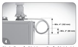
Attach silicone flexible tube or other flexible tube into a drain connection of the non-return valve. Create at least 4" (102 mm) diameter trap, pour water so that at least 3" (80 mm) water in the trap, and connect with a proper drain. All condensation must be drained and disposed of per local codes and requirements.
