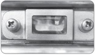
While the water heater is operating, inspect the main burner flames through the burner sight glass. The flames should be blue.
